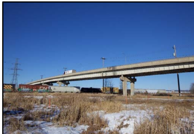
Figure 2. A long-span bridge in Thunder Bay, Ontario
