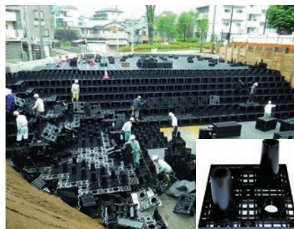
Units for rainwater storage and infiltration systems Photo : Joto Lyprone Co., Ltd.
