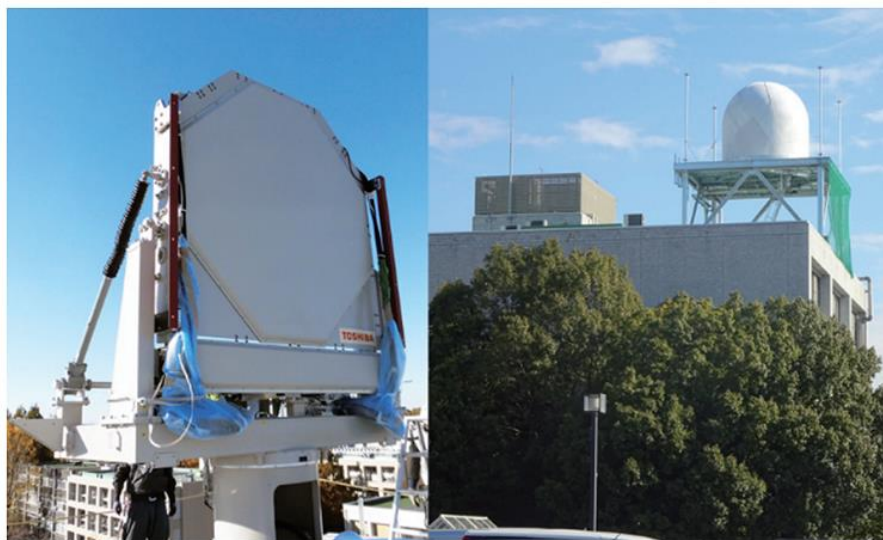
Fig. 4. MP-PAWR antenna (left) and the radome of MP-PAWR installed at Saitama University (right).
