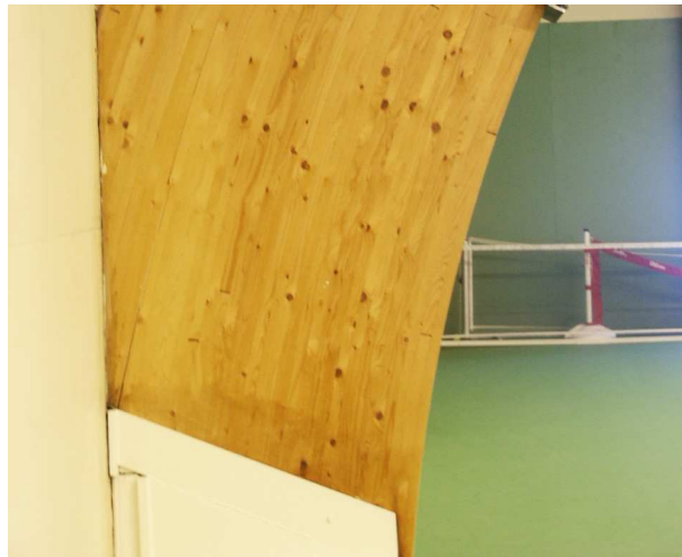
Figure 20. Arched column with steel parts (in white).
