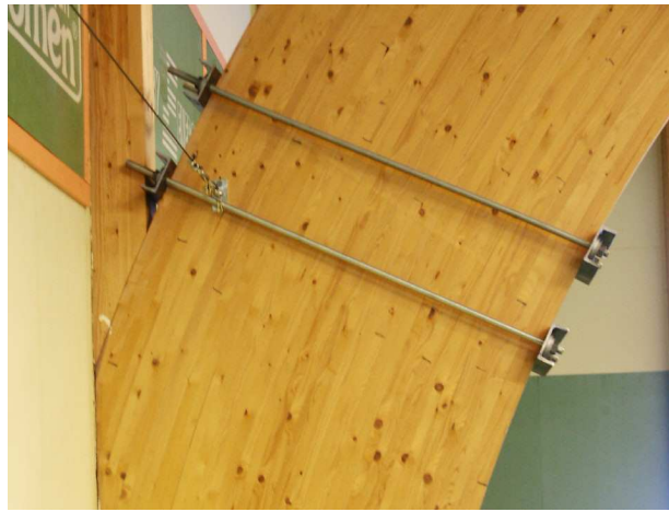
Figure 22. Temporary steel fixings attached to the column.
