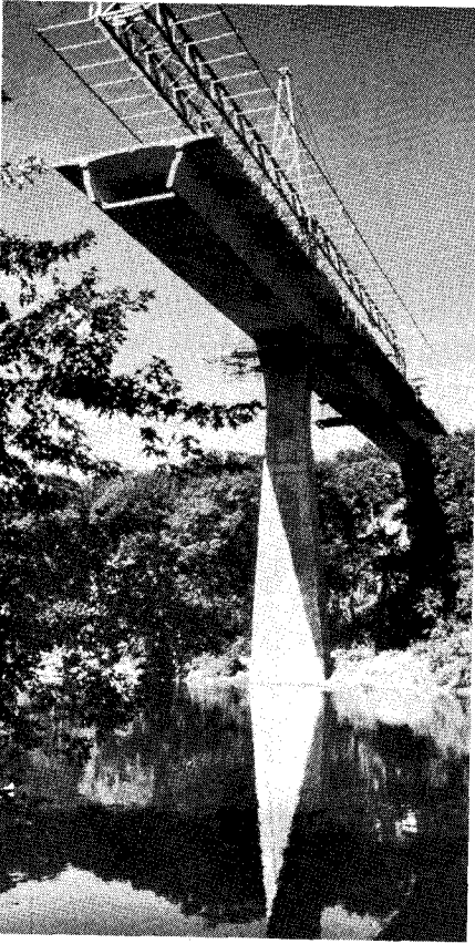
Fig. 8a. Kishwaukee River Bridge near Rockford, Illinois.
