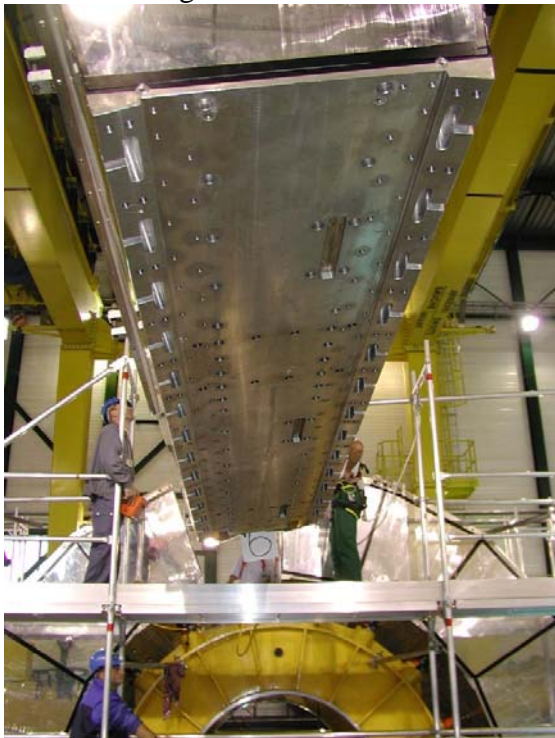
Installing the final wedge (18/18) of one HCAL half-barrel
