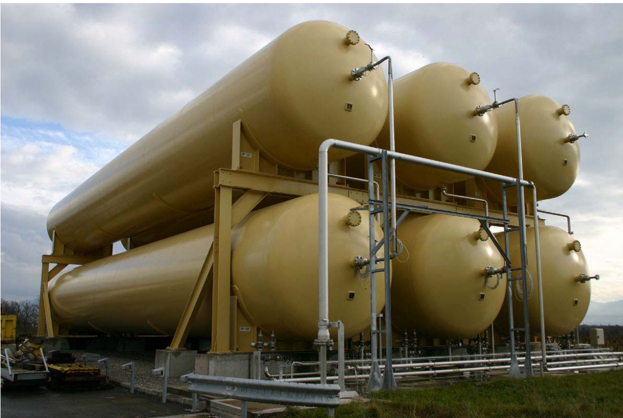
The cylinders that will contain the gaseous helium for the CMS/LHC cryogenic systems
