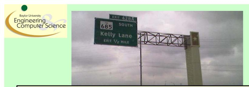
TX HWY 130 Sign Supports – Note the use of Pratt Truss construction
