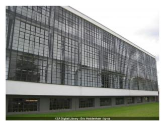
Figure 2. Glass curtain wall of the Bauhaus Dessau, 1926 [6].
