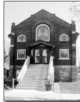
Lets insure the preservation of this wonderful building.
