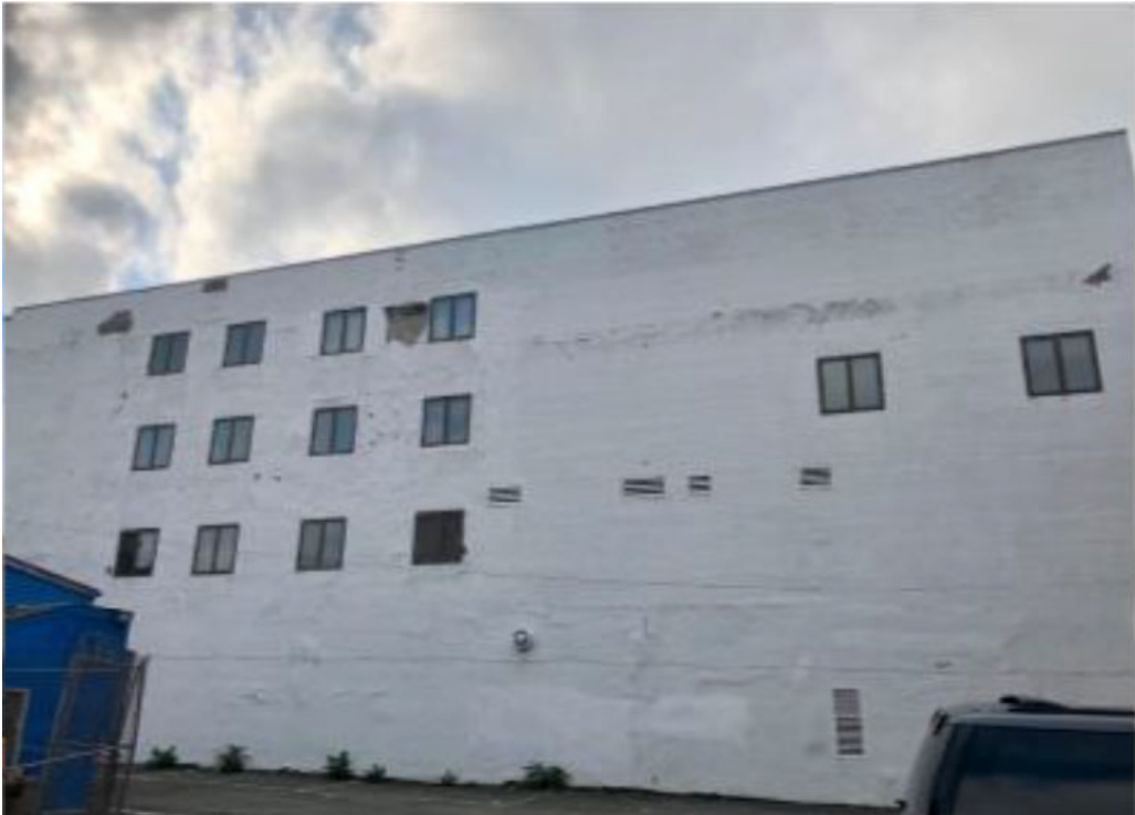
Figure 2: Building Side View
