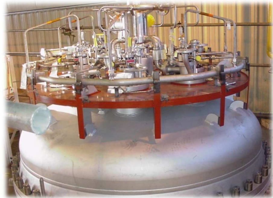
Final assembly of combustion chambers
