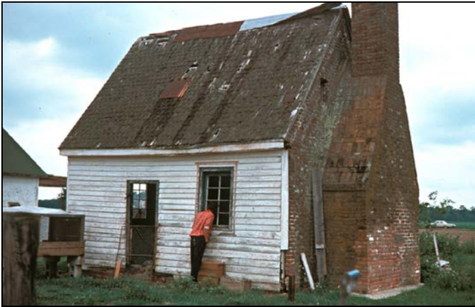
Figure 3. Preliminary field investigations of Pear Valley, Northampton County, Virginia, 1975 (Carl Lounsbury)
