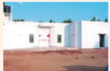
i-flex funded the development of infrastructure for Kutumba, a home for differently-abled and abandoned children.
