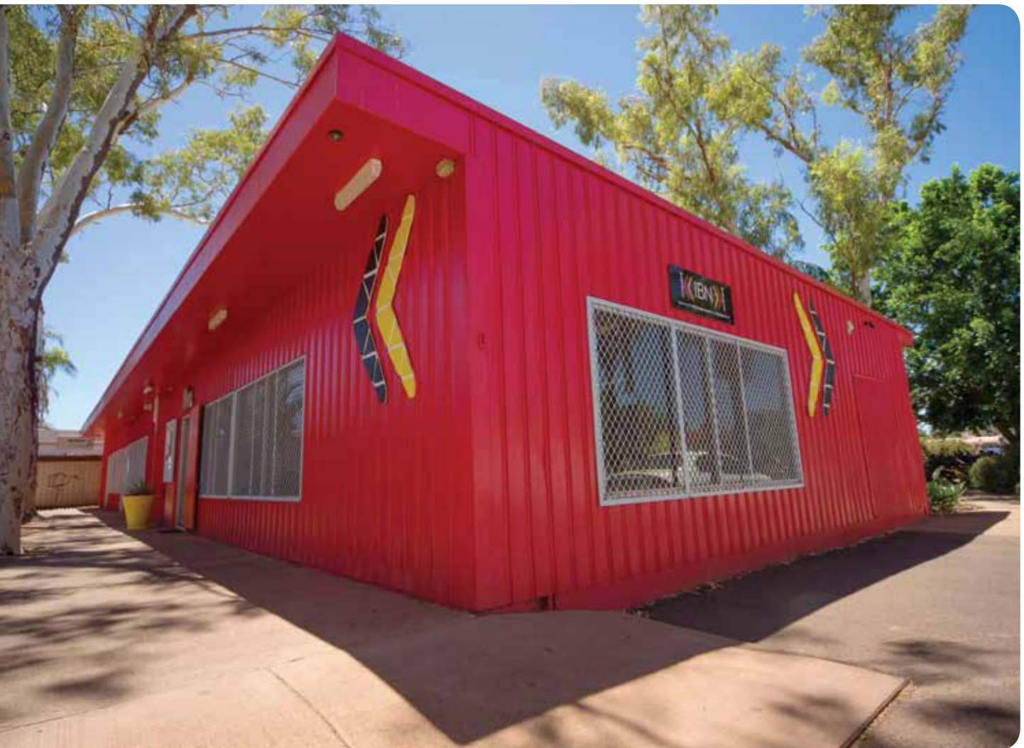
The new Tom Price office on Stadium Road.
