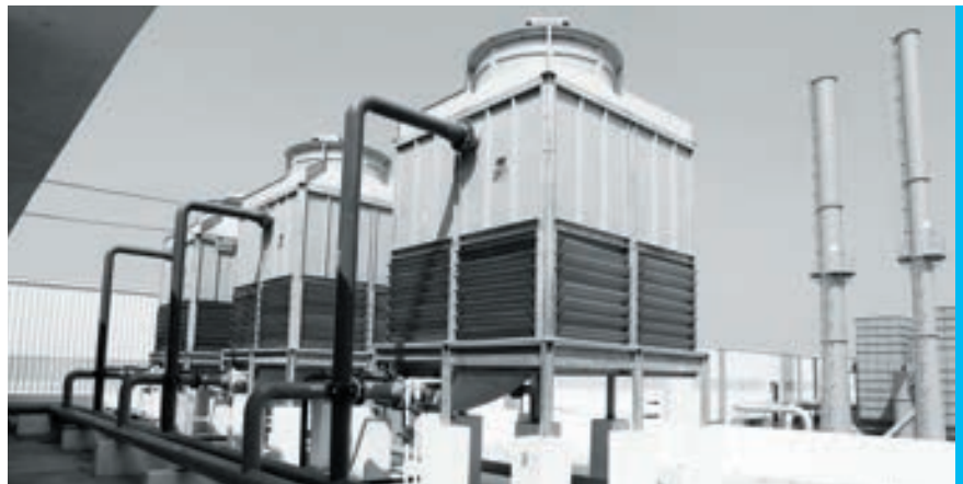
Chilling plant cooling towers
