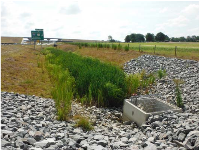
Stormwater basin east of mitigation site
