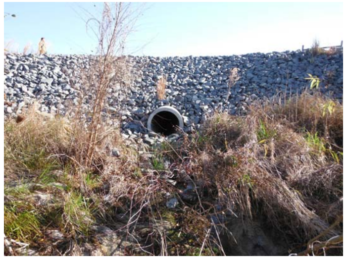
Stormwater outlet pipe into mitigation site
