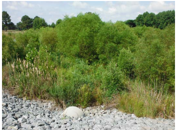
Stormwater outlet pipe into mitigation site
