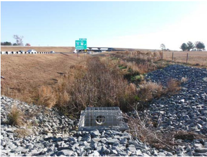
Stormwater basin east of mitigation site
