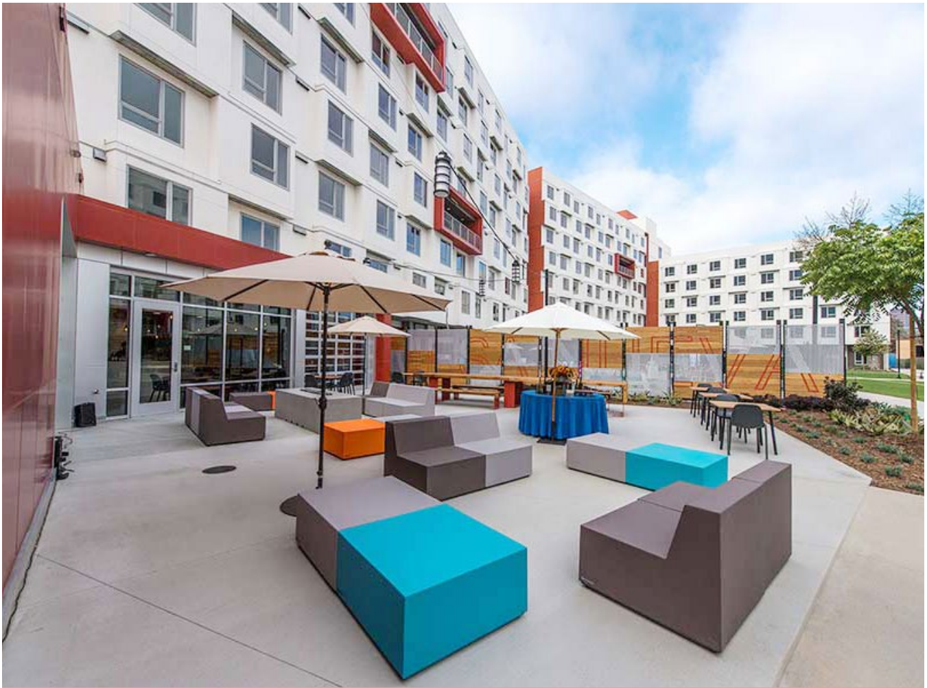
UC San Diego's newest housing project, Mesa Nueva, received the San Diego Gas and Electric (SDG&E) / Savings by Design Energy Efficiency and Integration Award in late 2018 and is a LEED Gold project. Credit: Rhett Miller
