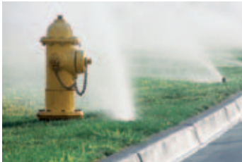
American Water fire hydrant
