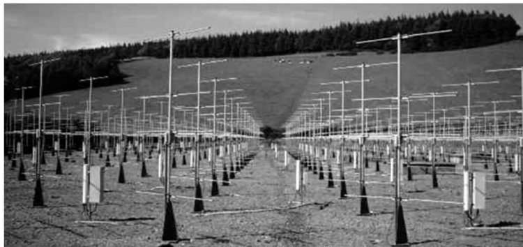
Figure 5-14. 46.5 MHz Wind Profile Radar in UK
