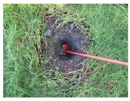
3. Start the anchor by hand, screwing it into the soil until it "bites" and starts pulling itself in. In stiff soils, some downward pressure will be needed. 4. Hold anchor at an angle so that the eye points to the guy attachment point on the tower. The picture shows axe handle inplace in the screw anchor eye. The axe handle acts as a lever for turning the anchor.
