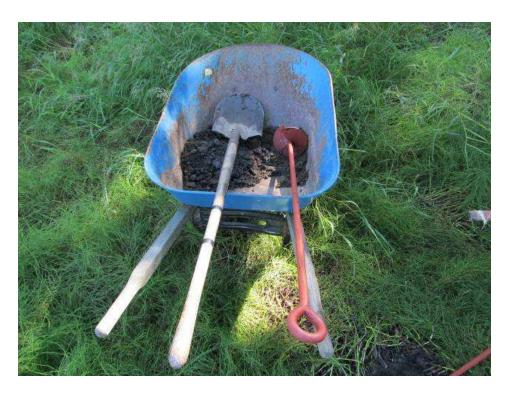
1. To start installation, gather the tools, a shovel and axe handle (not shown), and screw anchors. The screw anchor shown on the right side in the wheel barrow has a 48 in long by 5/8 in diameter shaft with 6 in auger on one end and a single eye on the other. 2. Dig a shallow starter hole, breaking through upper peat and roots. Picture shows the working end of anchor (the auger) ready to be inserted in starter hole.
