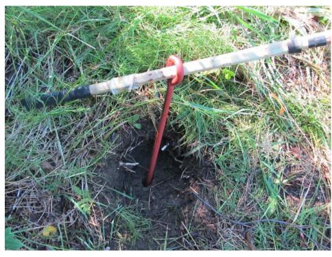
5. Stop every once in a while to rest and admire your hard work. The axe handle used to turn the anchor is shown inplace in the anchor eye. 6. Screw in the anchor until the eye is just above ground level. The axe handle used here is a replacement handle made from fiberglass and fit perfectly through the eye
