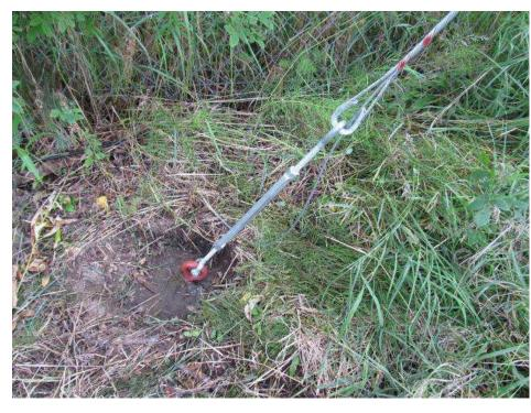
11. Another view of the anchor eye, turnbuckle, thimble, guy grip, and guy wire. After all guys are installed they are tensioned by adjusting the turnbuckle. 12. After the guys are tensioned, the excess guy wire is threaded through the turnbuckle and anchor eye to prevent the turnbuckle from turning on its own. It is then bonded to an earth electrode (for example, a ground rod).
