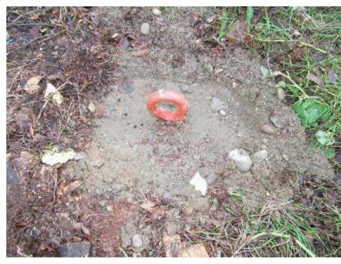
7. Complete the anchor installation by backfilling the starter hole and tamping the soil.
