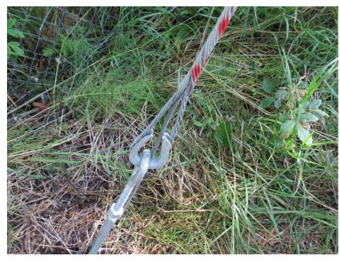
9. Another view of the guy grip showing the thimble and the upper end of a turnbuckle. The thimble protects the wire rope from chafing in the turnbuckle eye. The guy wire extends through the guy grip (see next step). 10. View of the guy grip, thimble and upper part of turnbuckle. The guy wire is long enough to be threaded through the turnbuckle, looped back and clamped. Turnbuckles are used at the anchor end of each guy to adjust tension.
