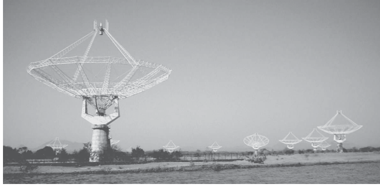
Fig. 1.2 A panoramic view of the Giant Metrewave Radio Telescope (GMRT), Pune, India, consisting of 30 fully-steerable parabolic dish antennas of 45 m diameter each spread over distances up to 25 km. 1 (Photograph by Mr. Pravin Raybole, Courtesy: GMRT, Pune, http://www.gmrt.ncra.tifr.res.in )
