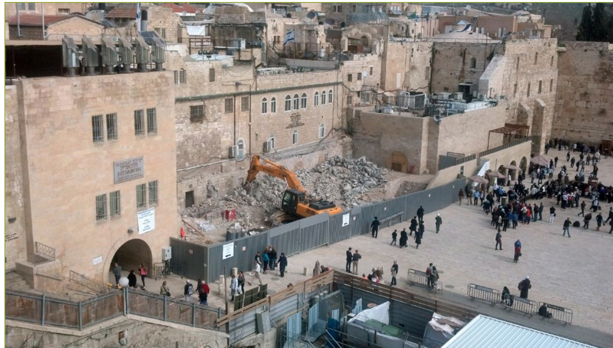
Demolition of the old Strauss building before the expansion
