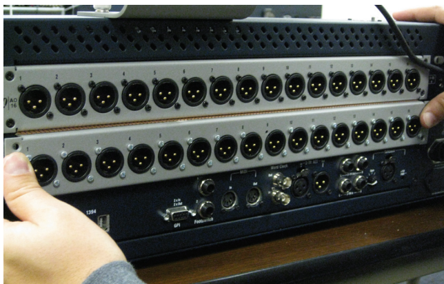
Installing the A016 Card
