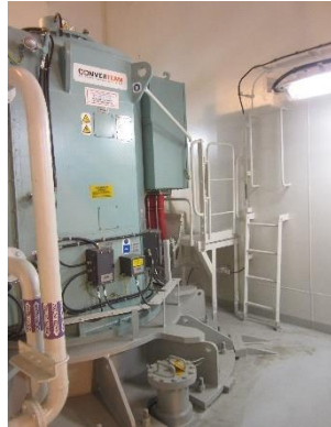
Blind flange replacement
