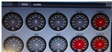
Leak test 165 bar
