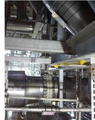
Heat exchanger isolation
