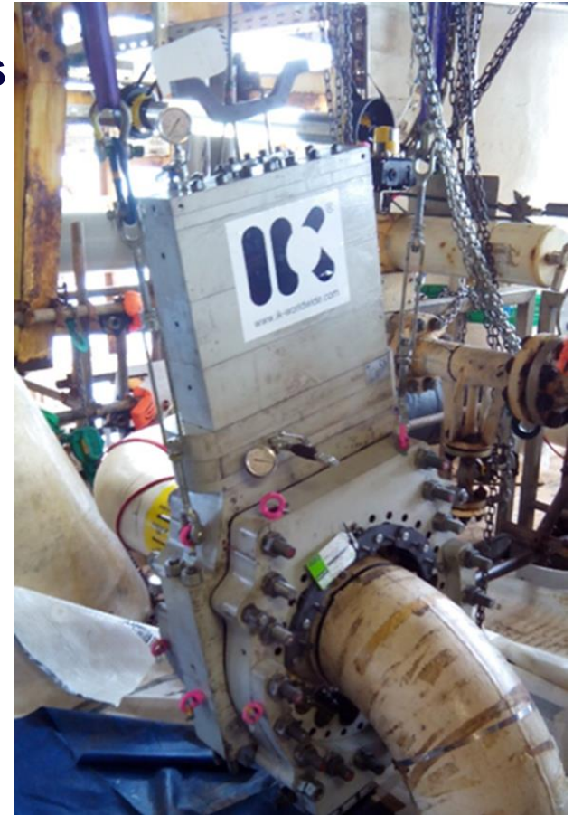
AOGV isolation complete
