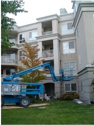
Figure 5.3.7 - Planning for access to building perimeter is essential if boom lifts are to be used. Capacity of parking garage roof slab and hard and soft landscaping features are critical considerations.
