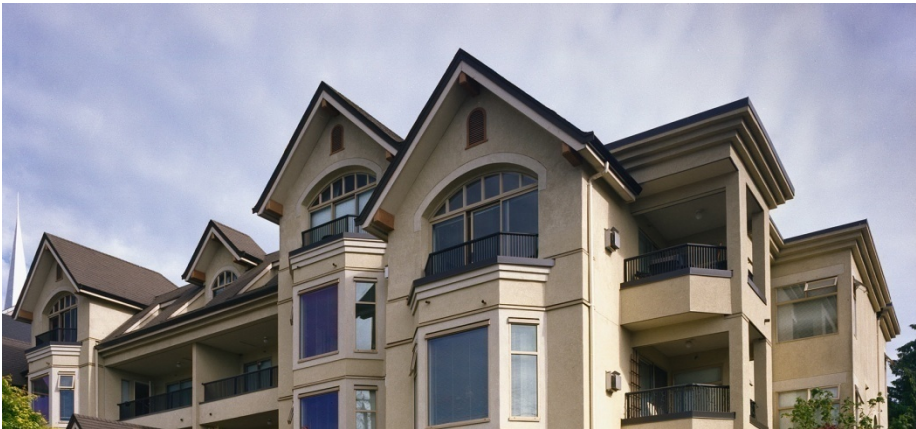
Figure 5.3.6 - Highly articulated roof line makes provision of roof anchors and use of suspended access equipment difficult.
