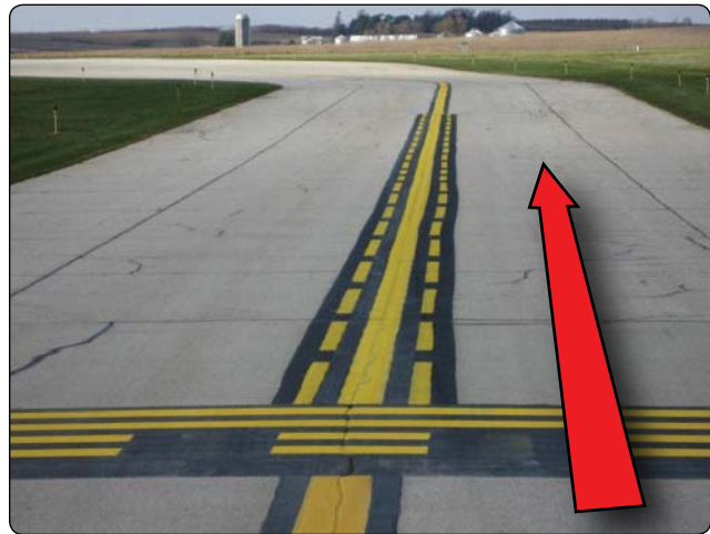
Figure 1-24. Runway holding position markings as seen when exiting the runway. When exiting the runway, no ATC clearance is required to cross.
