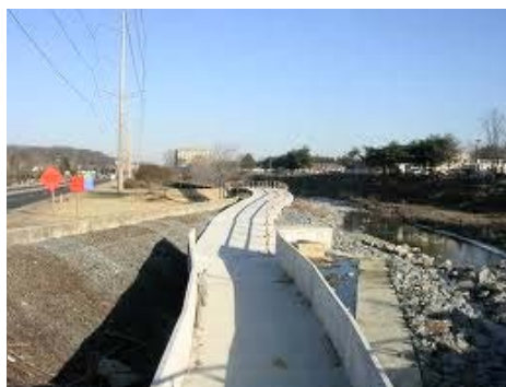
Figure 6-C.4. Channelized Section of Four Mile Run, Fairfax County, VA.
