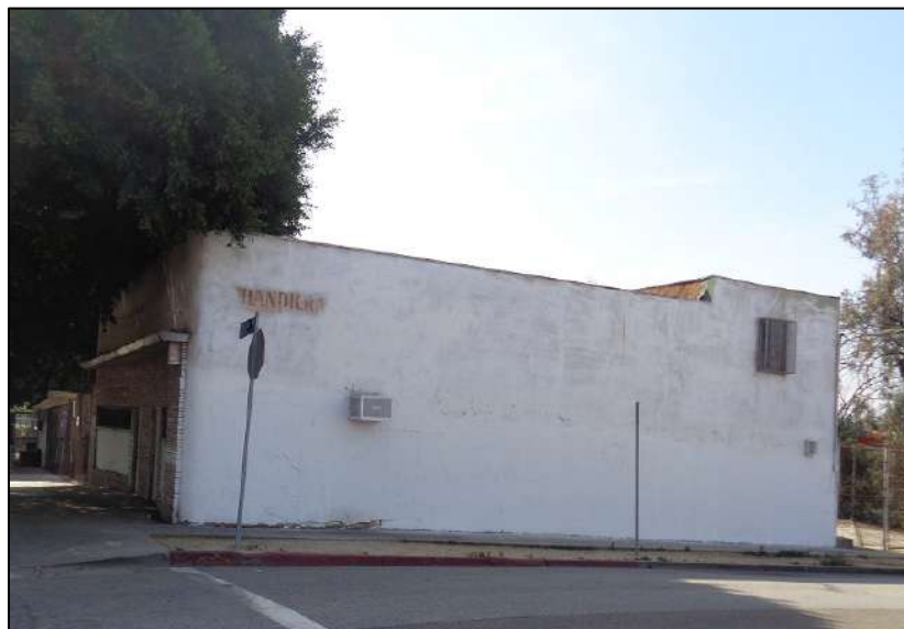
Figure 5: West elevation, camera facing southeast. ICF, 2018.
