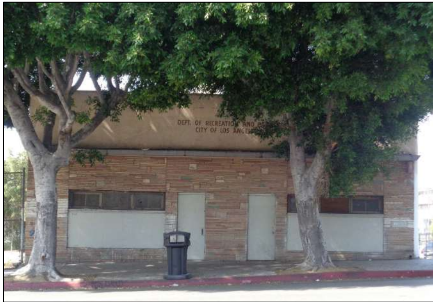
Figure 1: Primary elevation, detail, camera facing southwest. ICF, 2018.
