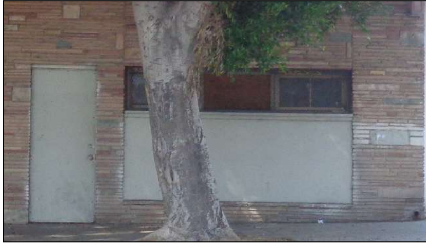
Figure 2: Primary elevation, detail showing west storefront, camera facing south west. ICF, 2018.
