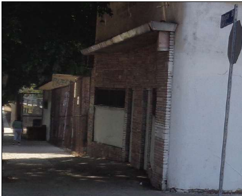
Figure 3: Primary elevation, detail showing canted walls, camera facing southeast. ICF, 2018.
