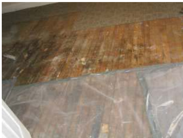
Typical Unit Flooring Under Carpet (moisture/water stains visible)
