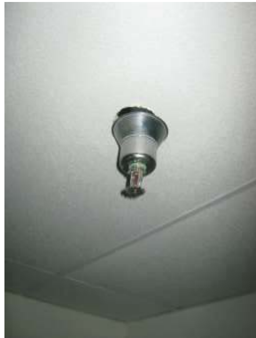
Typical Building Fire Sprinkler
