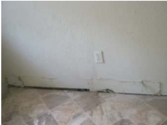
Water Stained Wall near Floor, 2 nd Floor Unit 1
