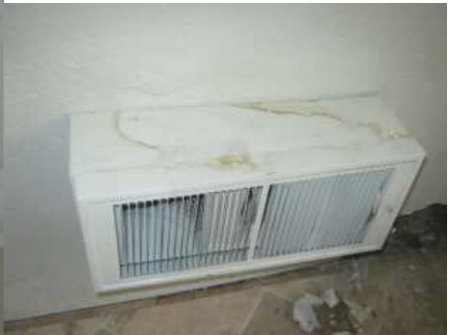
Water Stains on Ceiling & Vent Register, 2 nd Floor Unit
