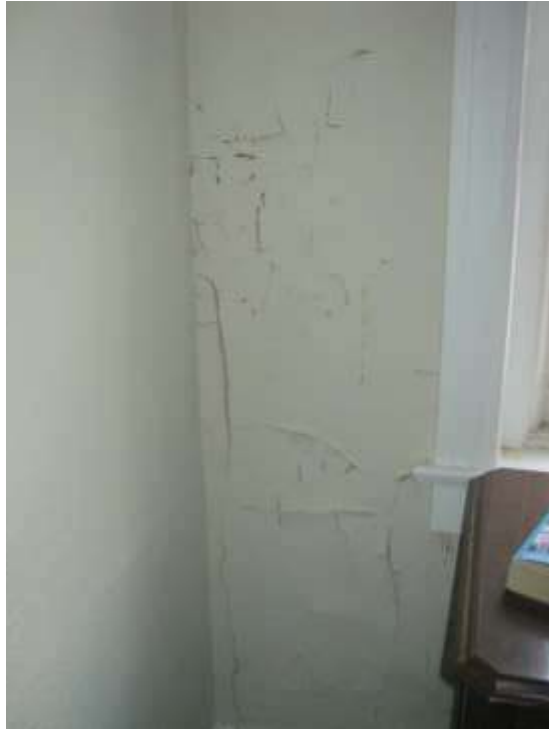
Cracked Plaster Walls, Unit 205 Living Room/Bedroom
