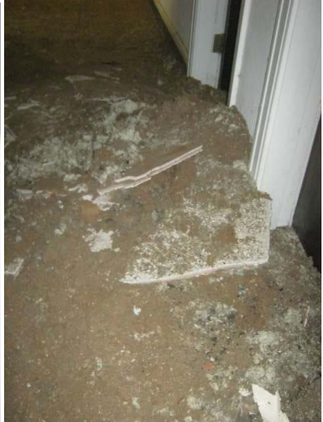
Fallen Ceiling Sheetrock/Insulation, 4 th Fl. Hallway
