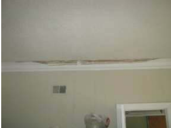
Water Stained Ceiling, 2 nd Floor Unit
