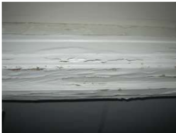
Water Stained Door Header, Unit 203 Bathroom
