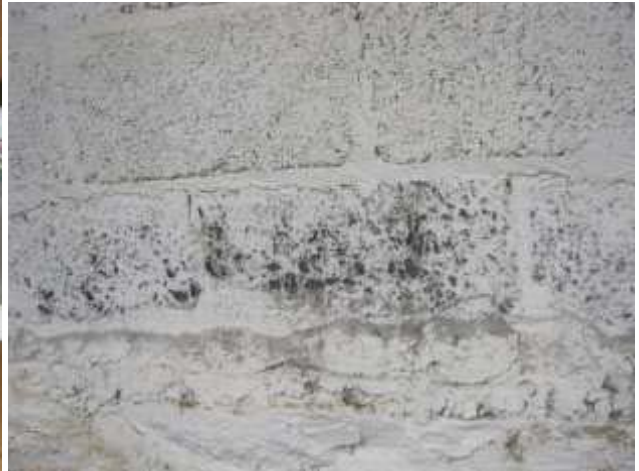
Visible Mold on Wall, NW Basement 1
