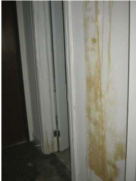
Water Stains, Unit 203 Main Hallway
