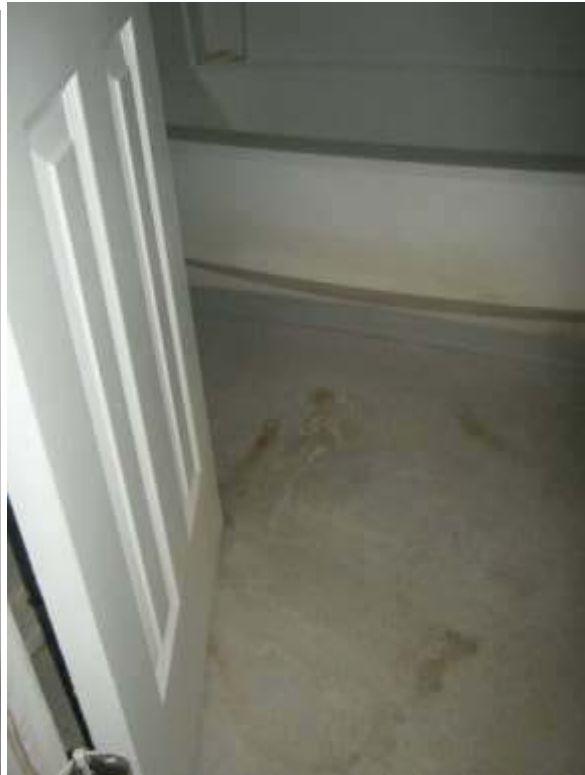
Water Stains, Unit 203 Bathroom Floor
