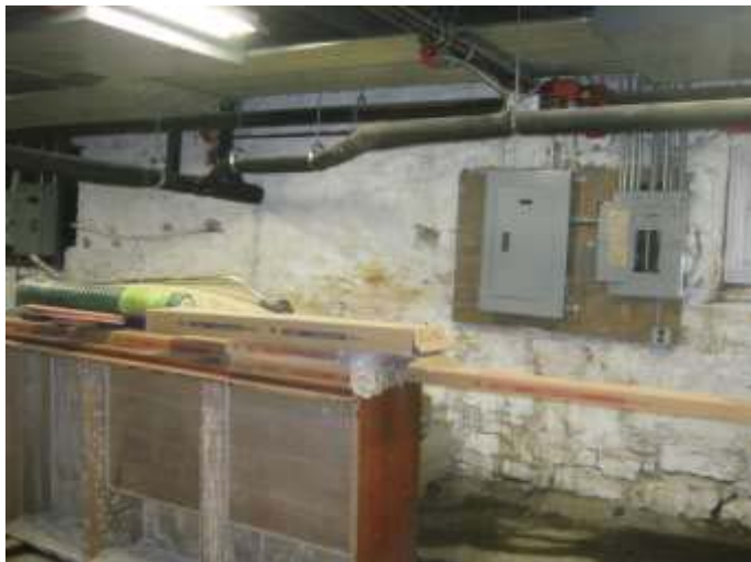
Basement Electrical Breaker Panels
