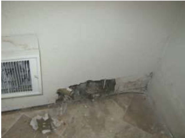
Water Stained Wall near Floor, 2 nd Floor Unit 2
