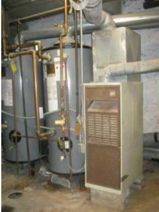
Hot Water Heaters & Furnace, Basement
