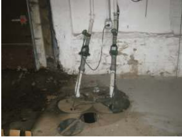
Sump Pump, East Loading Dock Area, Basement
