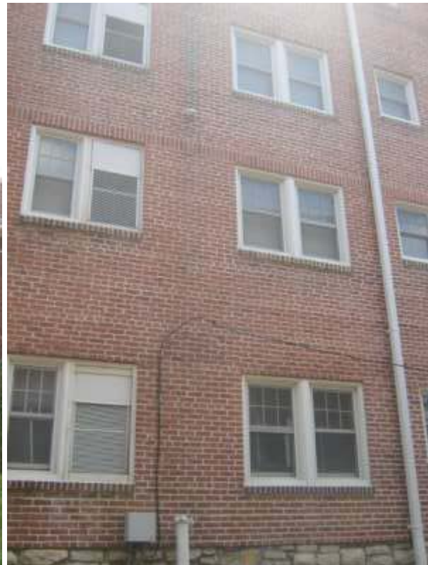
West Side Water Stain, Likely from Roof
