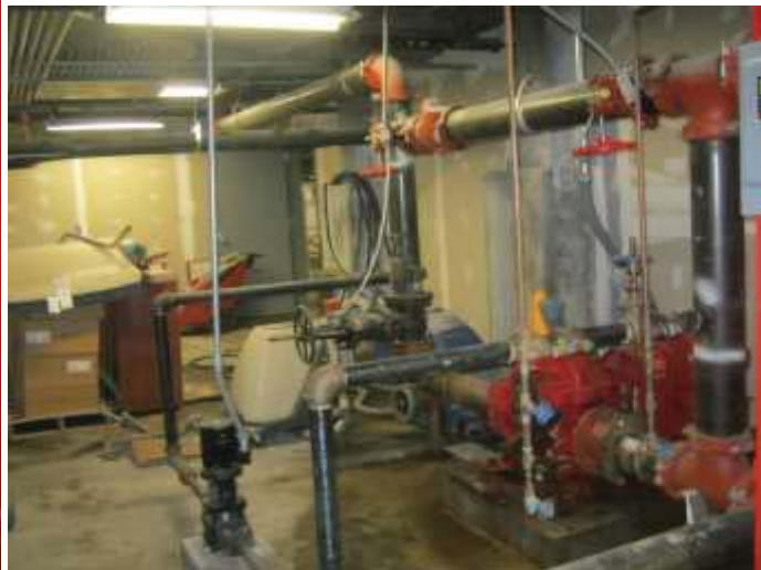
Fire Suppression System, Basement Utility Room
