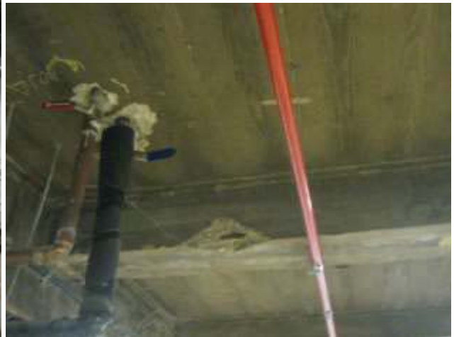
Hot & Cold Water Line Penetrations, Basement
