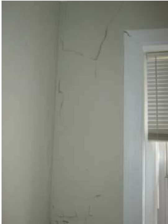
Cracked Plaster Walls, Unit 205 Living Room/Bedroom
