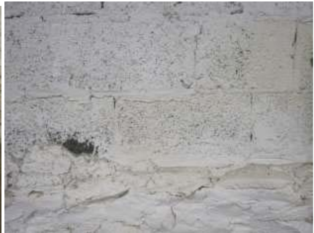
Visible Mold on Wall, NW Basement 2
