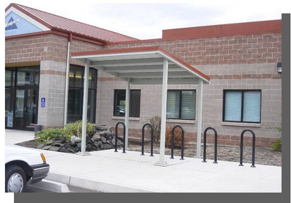
U-locks with shelter installed near a building entrance.
