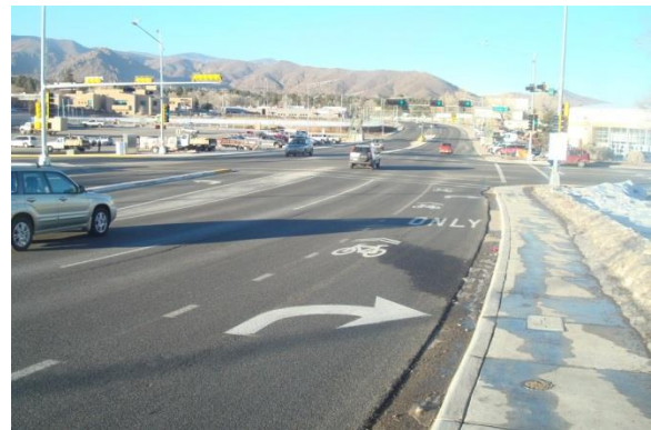
SLM Placed within Right Turn Lane
