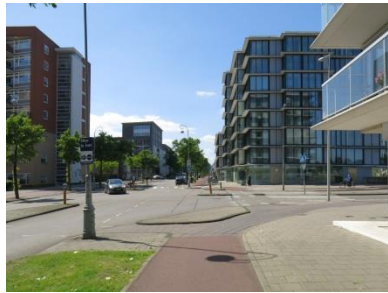
Corner Deflection Island
