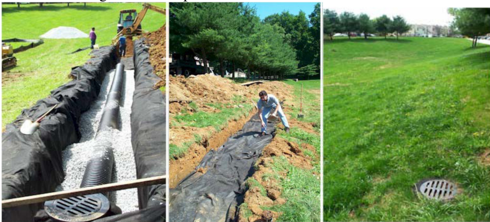
Figure 3: Example of Infiltration Trench Installation
