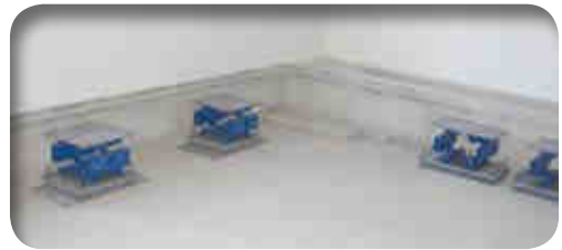
Protective suspension of mass-bed in laboratory
