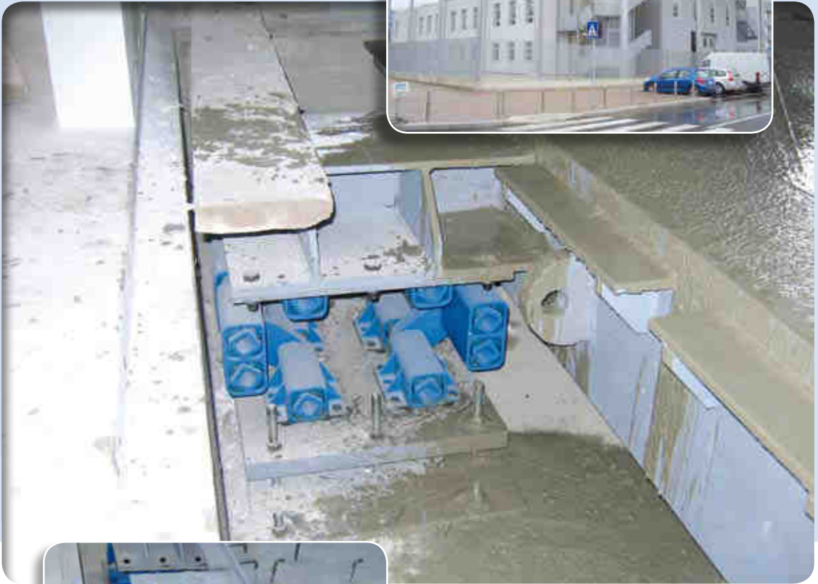
Protective suspension of mass-bed in laboratory
