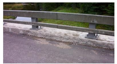
Figure 1. An Example of Premature Concrete Deterioration on an MTO NWR Project (Thunder Creek Bridge, MTO Site No. 41S-060)
