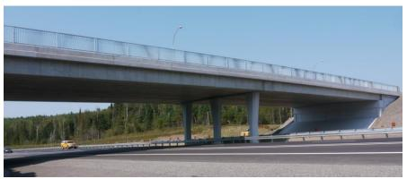
Figure 7. UHPC Pier Column Shells and Recessed UHPC Inverted T Pier Cap
