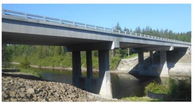
Figure 4. Adjacent Box Girder Bridge (Black River Bridge, MTO Site No. 48E-026)
