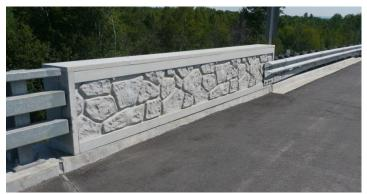
Figure 8. UHPC Barrier Endwall Treatment
