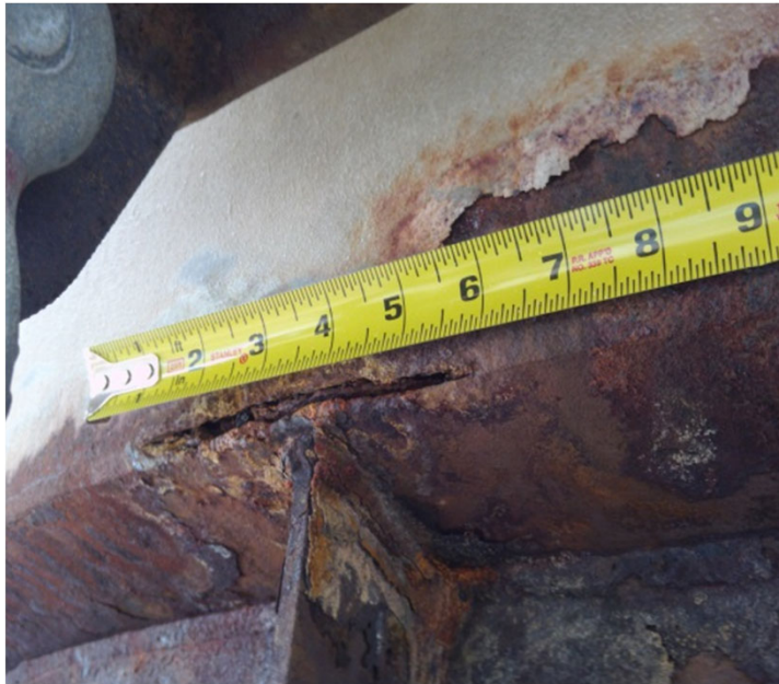
Observed Cracking
