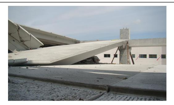
Figure 2. Collapsed Precast Double Tee Beams
