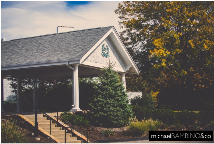
South Entrance—closest to restaurant
