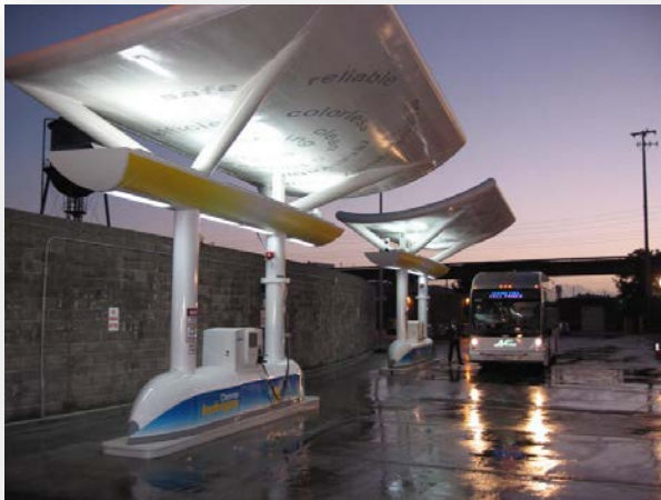
AC Transit – Reformer
