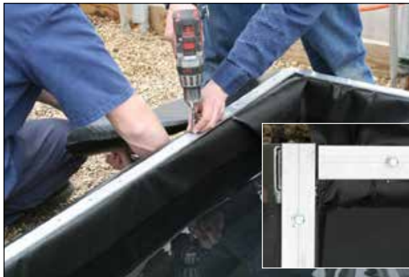
5. Continue attaching straps to the frame until the entire perimeter of the bed liner is secure.
