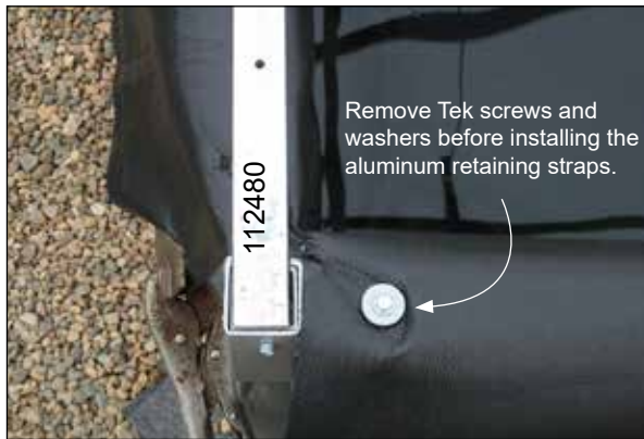
2. Align strap with end of frame and attach using the FA4472B Tek screw.
