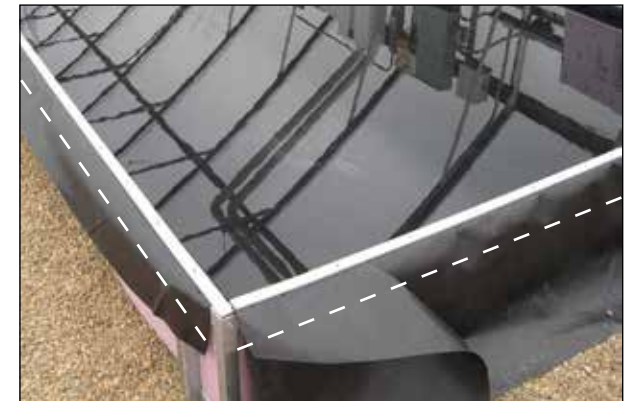
6. Using a utility knife or scissors, remove excess bed liner material. Allow 2"-3" to remain below the edge of the retaining strap.
