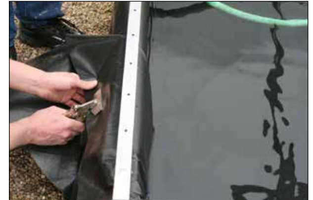
3. Grip edge of bed liner with duck-bill locking pliers or similar tool.
