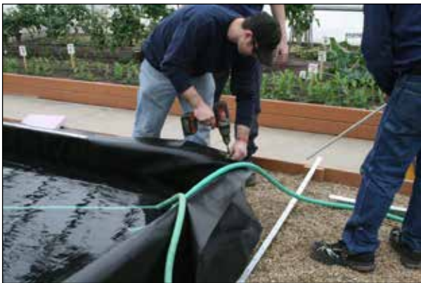
1. Begin at a corner and remove the Tek screw and washer to install first prepared strap.
