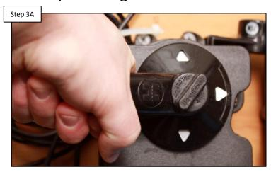
Verify the pump is running & valves are positioned so the flow switch is receiving water. IF the pump is not ON or the valve are not correctly set, resolve that first, then recheck. IF correct go to step 3B.
