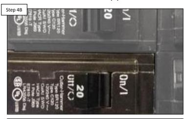
Verify the breaker, suppling the AquaRite power is in the full ON position. IF unsure OR breaker is ON, please contact service for further assistance (908) 355-7995 OR follow the link included below.
