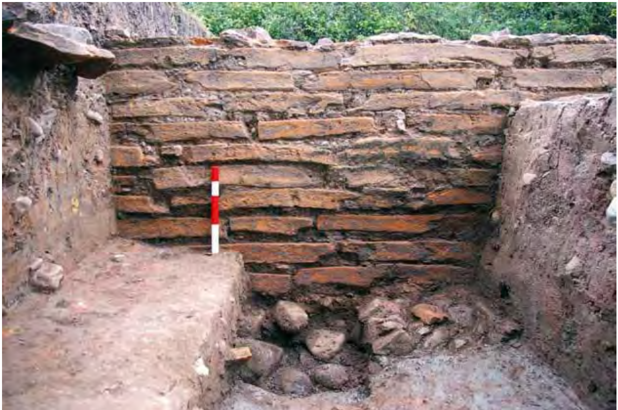
Fig. 14. West face of tegula wall [115] and underlying cobbled foundations (190)
