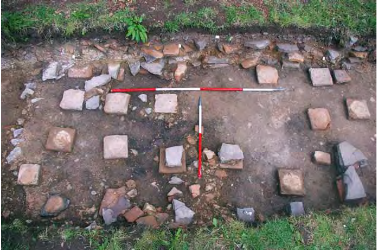
Fig. 68. Hypocaust in room 7.2 showing bases of pilae (718) on concrete bedding (714). Photograph taken from south
