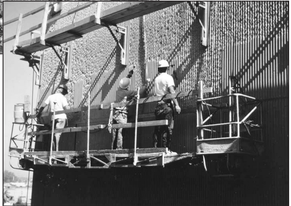
Figure 8-7. Fractured rib texture being developed
