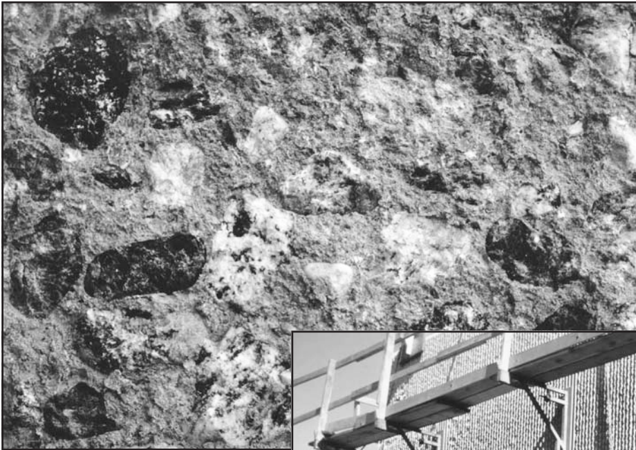
Figure 8-6. Bush-hammered surface
