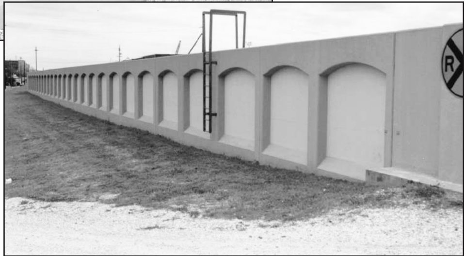
Figure 11-2. Painting of concrete highlights arches in floodwall
