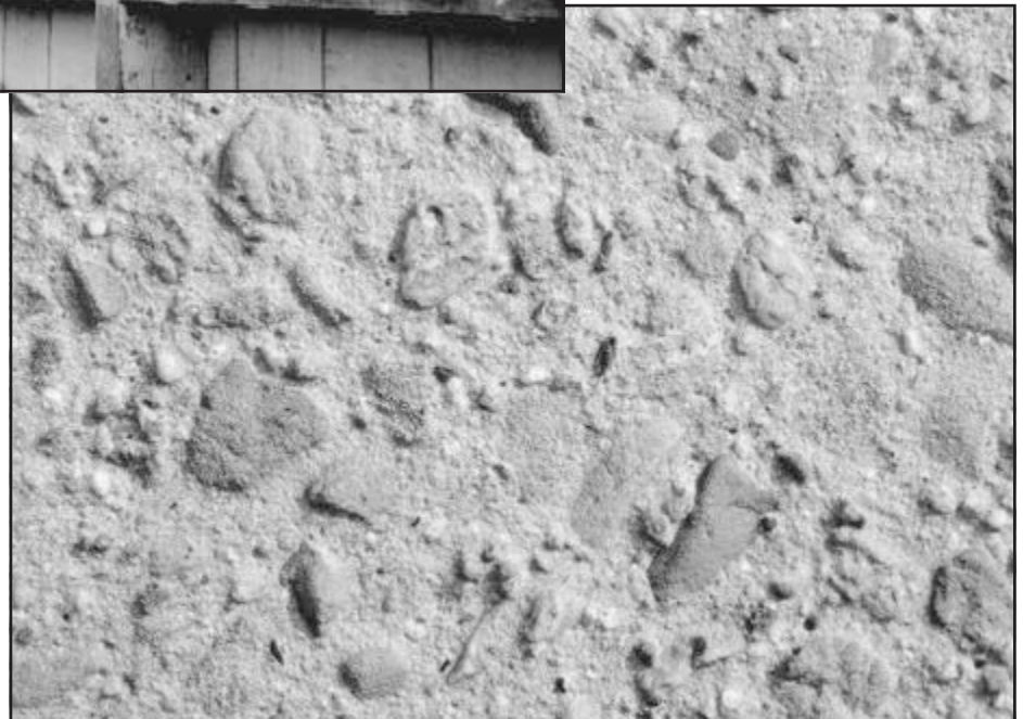
Figure 3-2. Textured finish by sandblasting
