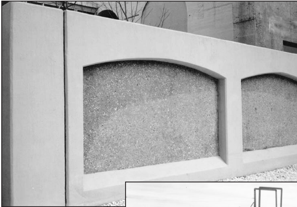
Figure 11-1. Architectural arch design in flood wall
