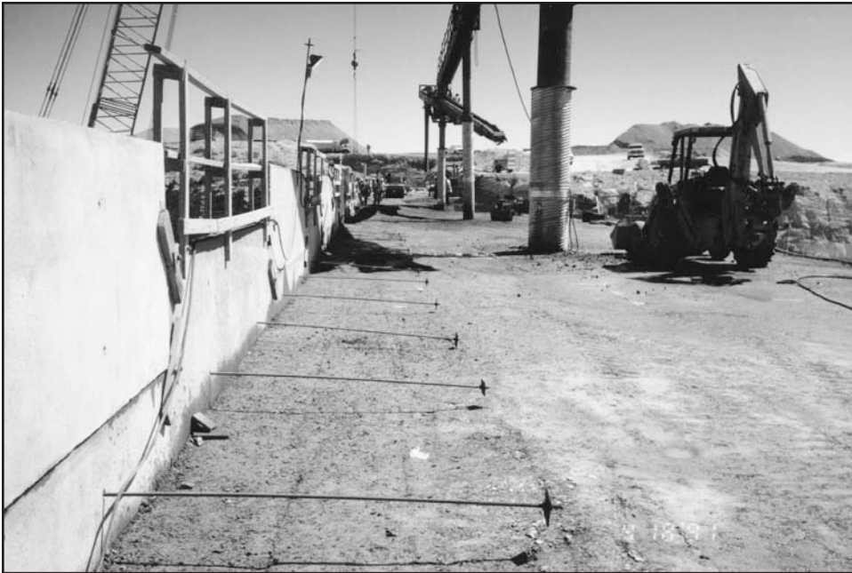
Figure 11-5. Form anchors in RCC placement
