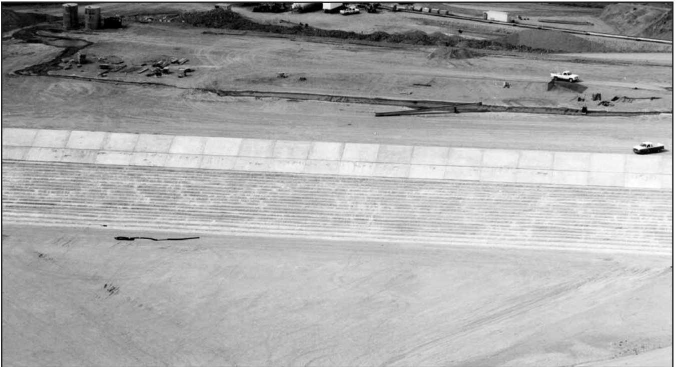
Figure 11-6. Step placement for RCC provides a natural bedded appearance
