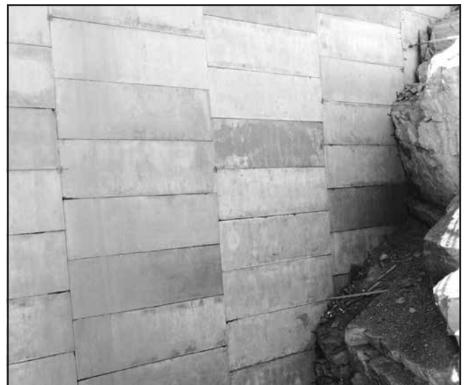
Figure 11-4. Precast concrete forms remain in place in RCC placement
