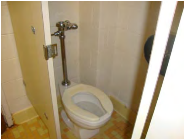
Figure 6.2: Typical Water Closet in Suite Bathrooms
