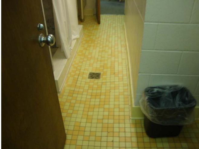
Figure 3.4: Typical Nonconforming Bathroom Hall
