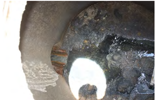
Sewer Manhole at Belk Hall
