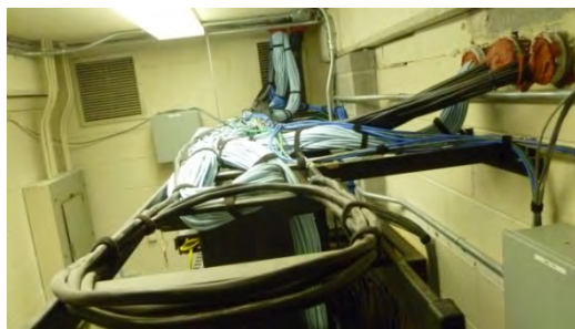
Figure 5.11 Typical horizontal cabling at MDF
