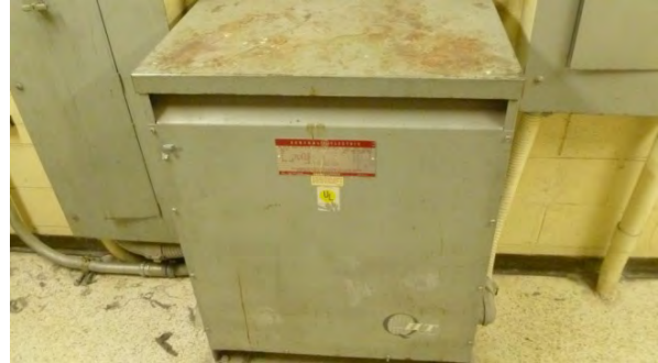
Figure 5.7 Typical 112.5 kVA Step-Down Transformer
