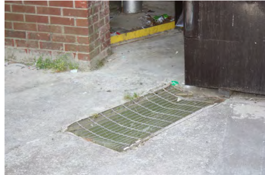
Drain at dumpster
