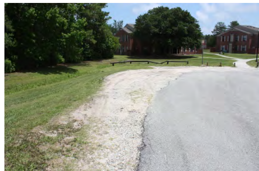
Rear Access Road
