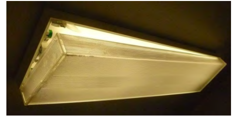
Figure 5.2 Belk Hall Fixture with T8 Lamp System
