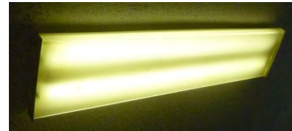
Figure 5.1 Graham-Hewlett Typical Fixture with T12 Lamp system
