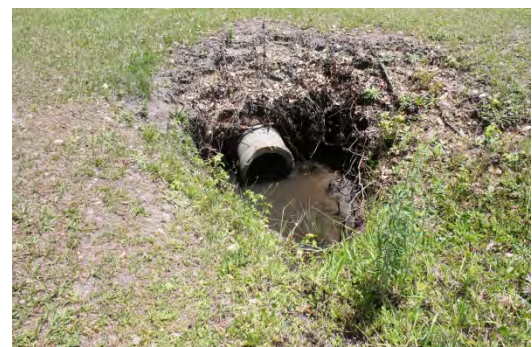
Inlet pipe at ditch
