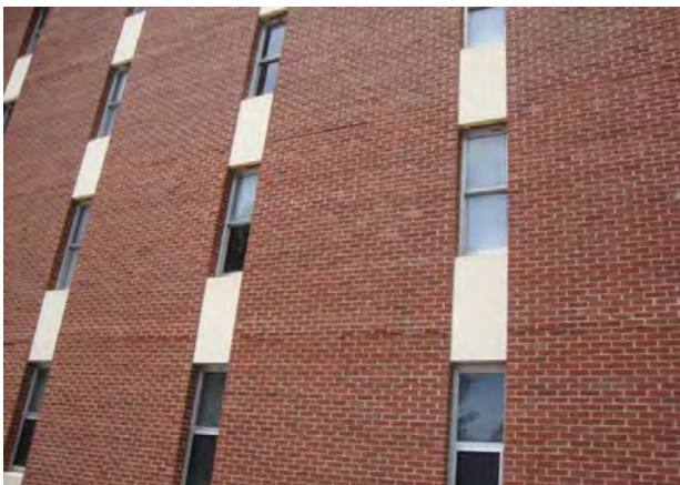
Figure 3.1: Hewlett Hall Exterior Face Brick
