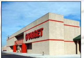
Project: Target T-2340 Location: Burnsville, MN, USA Precaster: Fabcon Inc. Technology: Versacore Sandwich Wall Panels Blockouts and Deadman Design using LECWall and spreadsheets for Precast insulated wall paneled Store.
