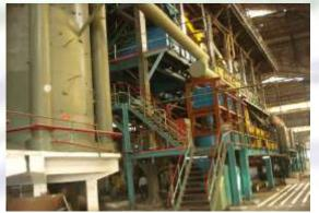
Project: Mayuge Sugar Factory Location: Jinja, Uganda Client: Saisidha Sugar Equipment & Engineering Co. Pvt. Ltd. Capacity: 2500 Tons per day Cost: Rs. 1000 Million Technology: Reinforced Cement Concrete and Steel Scope: Conceptualize, design, drawings, fabrication drawings and BOQ for 2500 TPD plant structures, foundations, machine foundations, client coordination, stability certificate.
