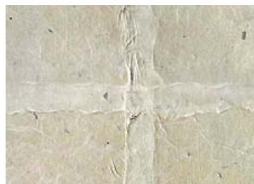
overlap installation (live edge)
