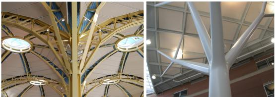
Fig. 2: Consider the case of these two "tree" structures. The structure for Reagan International Airport (left) uses more standard section types to create a very tactile aesthetic while the support at the right uses pipe and castings that have been carefully fabricated to support a high gloss finish. Two unique specifications were required.
