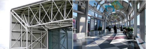
Fig. 1: Sainsbury Center by Foster (left) versus O'Hare International Airport by Murphy/Jahn (right). Sainsbury is rigorously modular where O'Hare begins to make more flexible use of a *family* of connection details.
