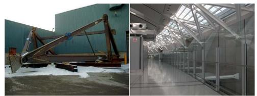
Fig. 4: The element at the left was the visual sample for the project. Given its size and expense, it was incorporated into the finished building. To find it on the right is akin to "Where's Waldo". Hence a cost and time saving that was worthwhile.
