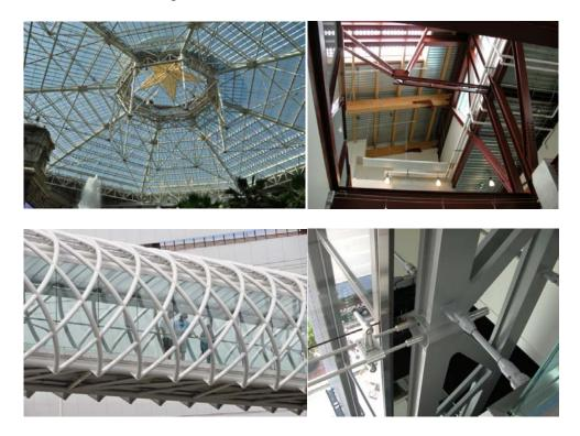
Fig. 3: The AESS Categories: (top left) AESS 1, (top right) AESS 2, (bottom left) AESS 3, bottom right (AESS 4). AESS 1 and 2 are located beyond 6 meters where AESS 3 and 4 are within view range and touch.
