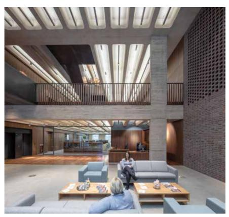
Environmental efficiency plays a key role in the design of Royal College of Pathologists building with exposed coffered concrete slabs used throughout the building to form part of the passive cooling strategy. By increasing the surface area of thermally active concrete, Bennetts Associates significantly improved the environmental efficiency of the building Photo courtesy Bennetts Associates
