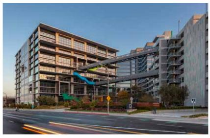
Dis-conditioning spaces by moving stairs outside relieves the need for heating and cooling them thus reducing operational energy. This move also creates a positive experience for building occupants by giving individual front doors for tenants occupying upper floors of office buildings. Photo courtesy Gensler
