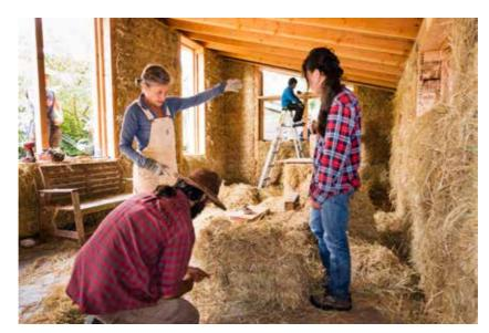
Constructing the exterior straw bale walls of house in California Photo: Edward Caldwell / courtesy Arkin Tilt
