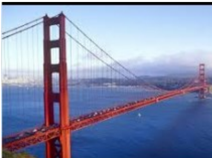
January 5, 1933 Begin Golden Gate Bridge Construction
