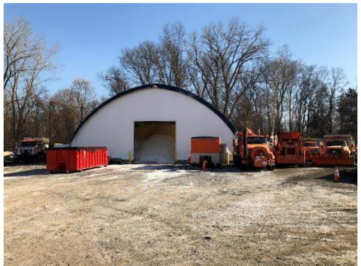
Salt storage shed
