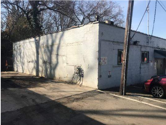
Exterior - Main office and garage building
