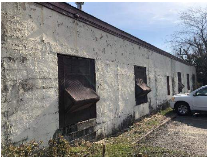
Exterior - Parking area on southern side of building
