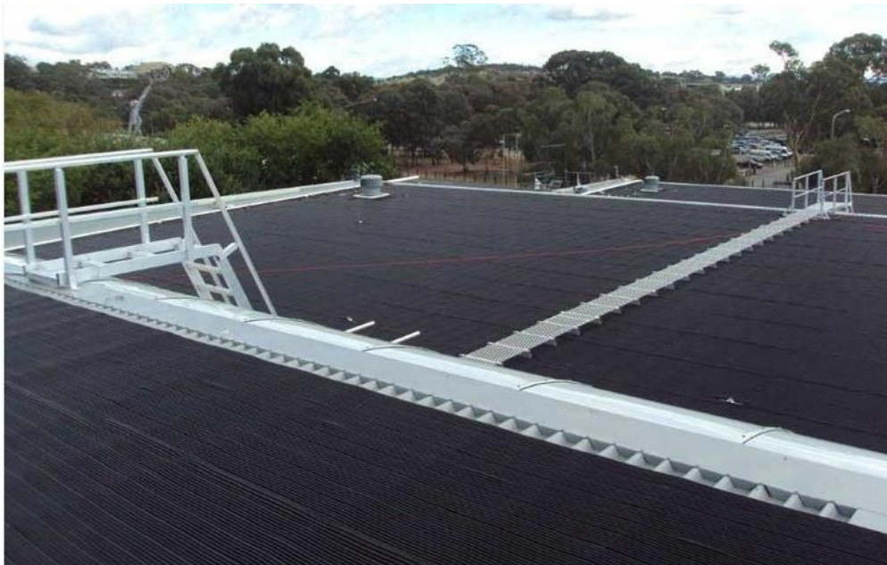
Figure 106: Unglazed collector for an indoor pool at the Australian Institute of Sport, Canberra. (Reproduced from Sunbather).
