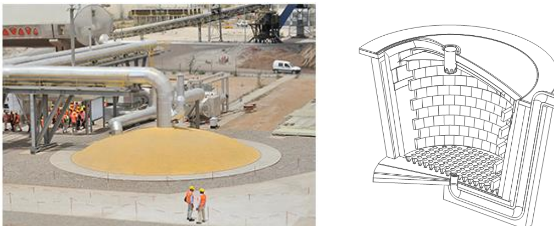
Figure 135: Packed bed thermal storage system. (Reproduced from Airlight Energy).
