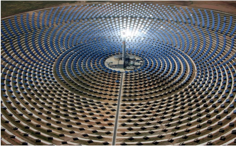
Figure 115: Aerial view of the Gemasolar solar tower plant in Spain, thermal capacity 400 MW th . (Image from Torresol Energy).
