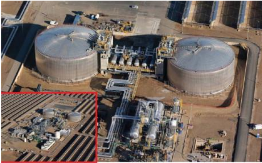
Figure 133: Image of a large-scale molten salt storage system used in a parabolic trough solar power plant. (Reproduced from Heliocsp).
