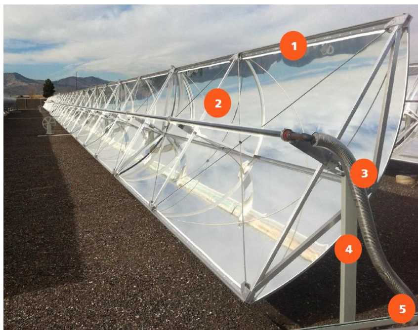
Figure 111: Parabolic trough collector construction, 1 Concentrator with aluminium or glass mirror, 2 Receiver tube, 3 Flexible coupling, 4 Pylons, 5 Header piping. (Figure from Abengoa).
