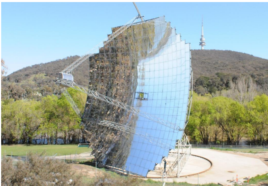
Figure 116: Australian National University's prototype 500m 2 paraboloidal dish concentrator (image K Lovegrove).
